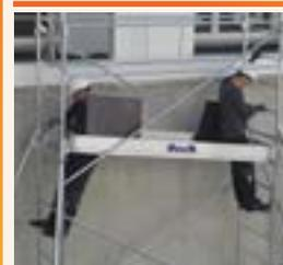
**INSTALLATION EN SÉCURITÉ DU PLANCHER.**
