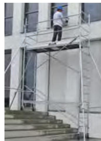
**INSTALLATION EN SÉCURITÉ DU PLANCHER.**
