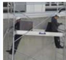
**INSTALLATION EN SÉCURITÉ DU PLANCHER**
